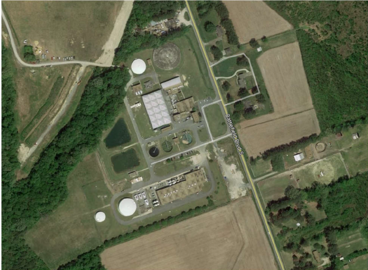
Figure 2. Northwest River Water Treatment Plant (NRWTP)
