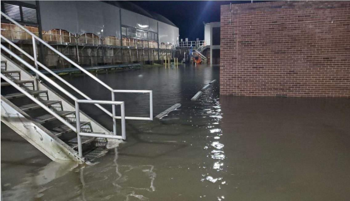
Area between Admin/Lab Building and Sedimentation Basins
