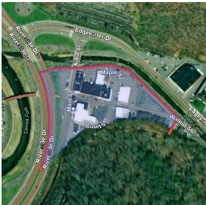
Figure 6-12: System and Area Protected by Grundy Levee System
