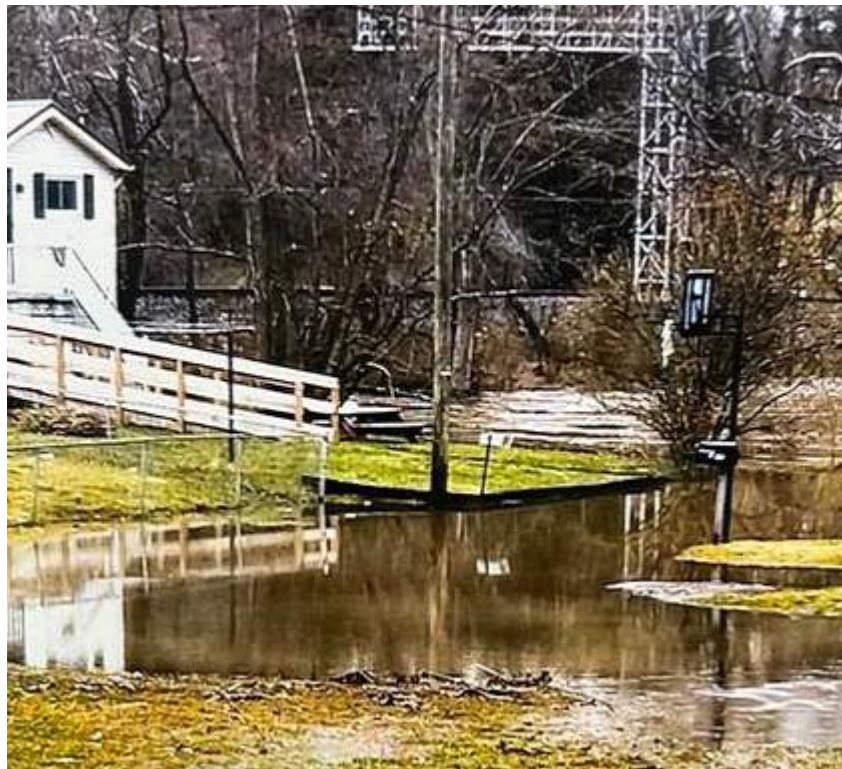
Figure 719: Flooding of Blacksburg Street
