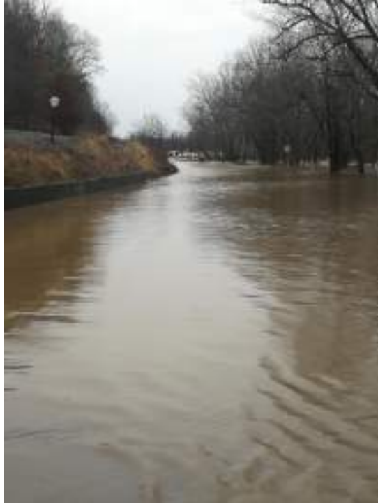
Figure 622: Route 67/Raven Road Inundated with Floodwaters on February 6, 2023
