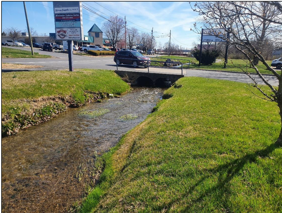
Photo 4. Culvert Crossing at Winchester Area SPCA
