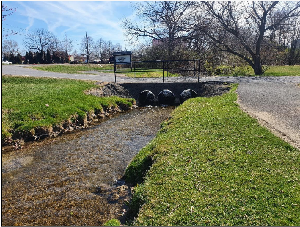
Photo 6. Culvert Crossing in close proximity to upstream SPCA Culvert Crossing
