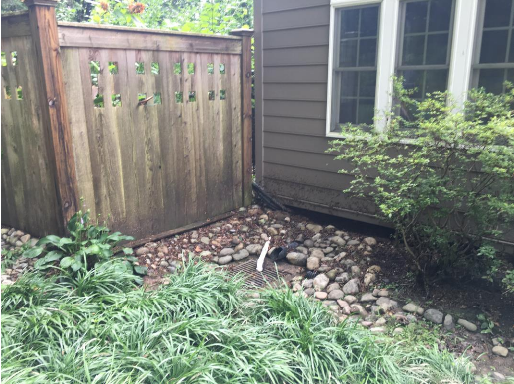
Figure 1: Post Flood Pictures
