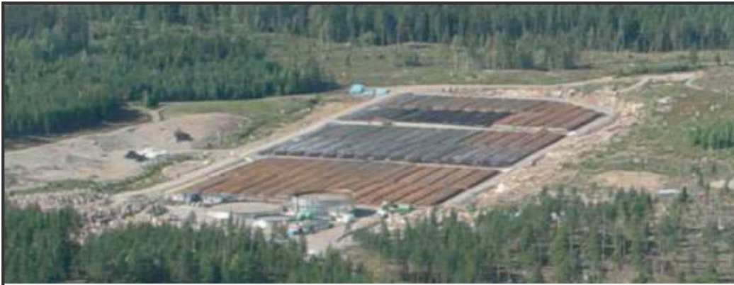
Figure 11. Geotube Disposal Method
