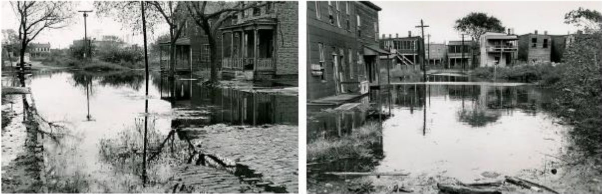
Tidal flooding on October 23, 1953, near Charlotte Street and Walke Street (NRHA)
