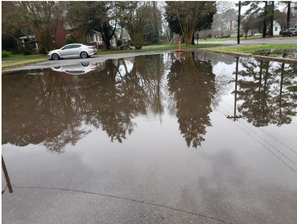
Photo 6: Flooding of a parking lot in the town of Nassawadox due to rainfall and inadequate drainage.
