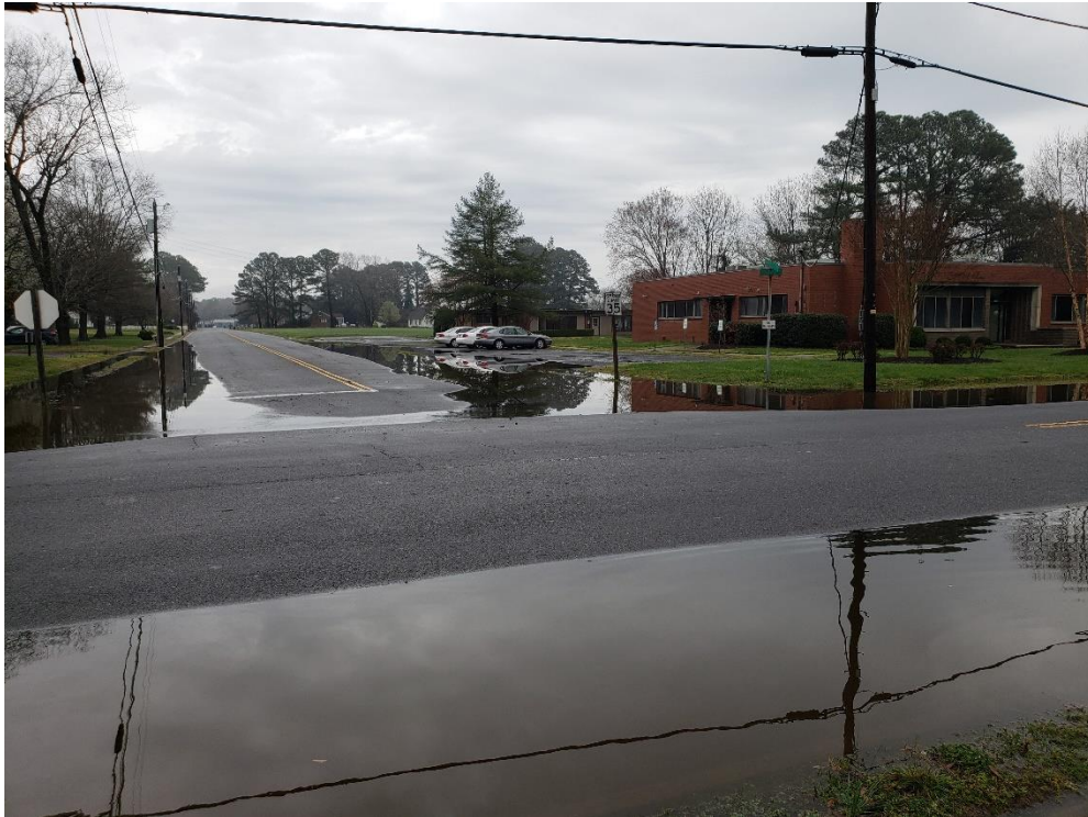
Photo 4: Flooding in the town of Nassawadox from rainfall and inadequate drainage.
