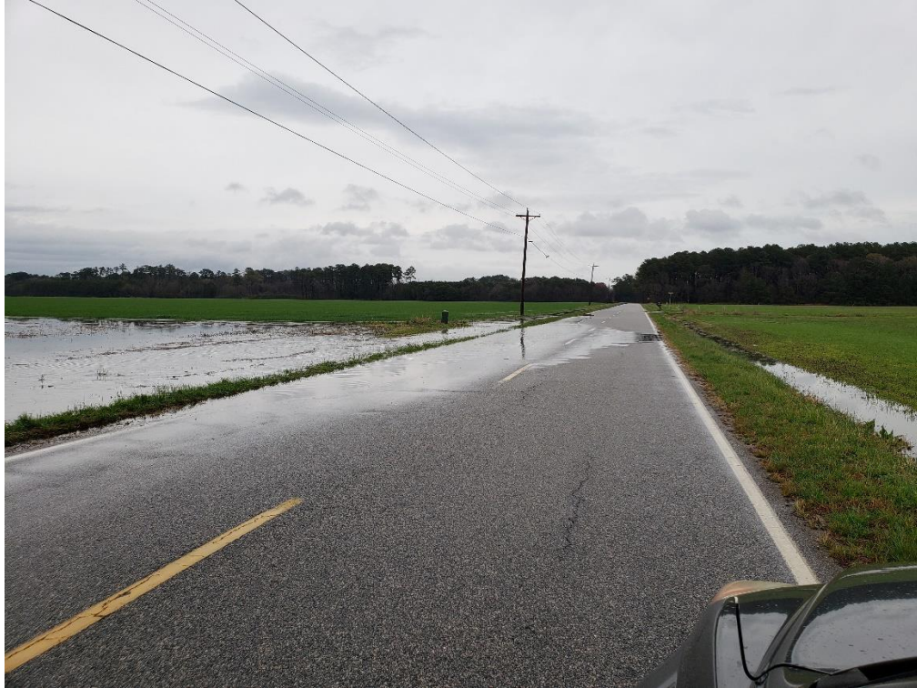
Photo 3: Flooding on Church Neck Road and adjacent farm fields from rainfall and inadequate drainage.
