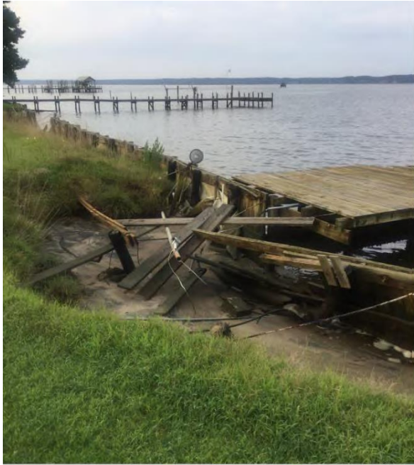
As the bulkhead failed the shoreline eroded the land away from the pier causing it to collapse.
