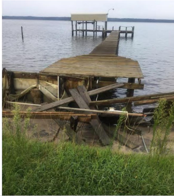
As the bulkhead failed the shoreline eroded the land away from the pier causing it to collapse.
