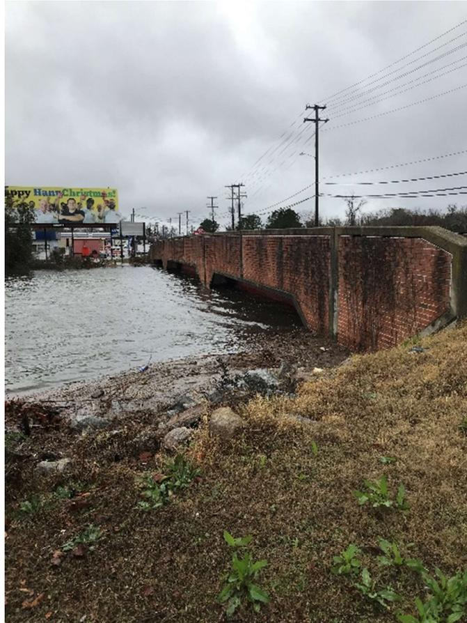
Floodwaters and Nansemond River Tides rise above the hydraulic opening of the Kimberly Bridge on Jan. 3, 2022, causing flooding of North Main Street (U.S. Route 32/U.S. 460 Business); resulted in extended road closures and traffic detours for several hours.
