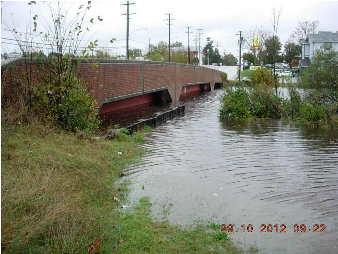
Floodwaters and Nansmond River Tides rise above the hydraulic opening of the Kimberly Bridge during Hurricane Sandy in October 2012 causing flooding of North Main Street (U.S. Route 32/U.S. 460 Business), resulting in extended road closures and traffic detours for several hours.
