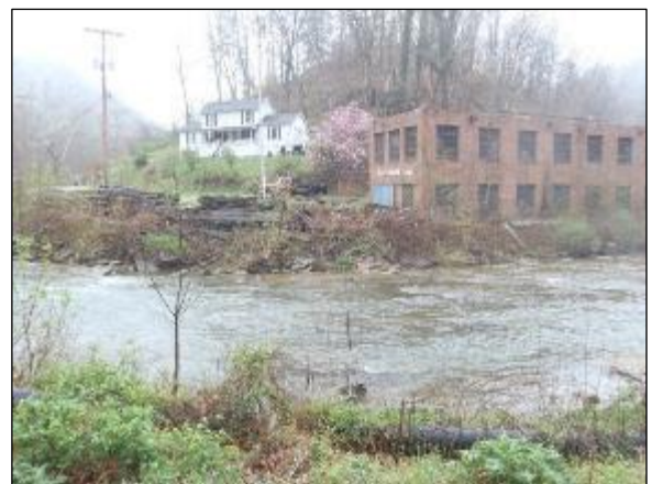
Image 2. Cedar Bluff Woolen Mill building.
