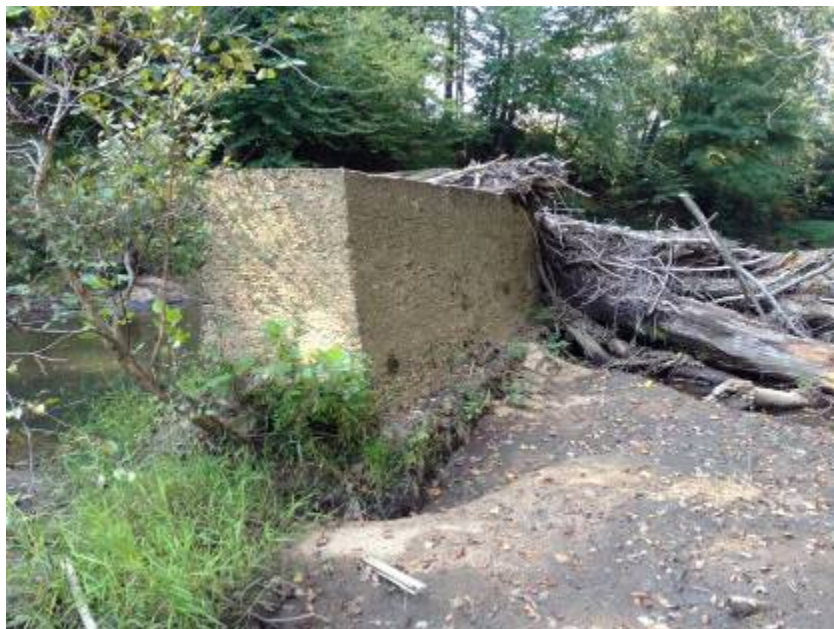
Image 11: Old Bridge footing at confluence of Flat Rock Creek
