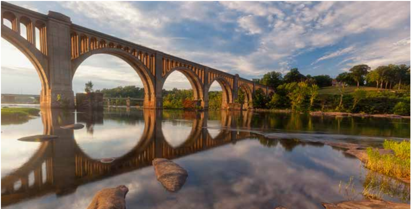
James River Railroad Bridge, Richmond | David Nguyen
