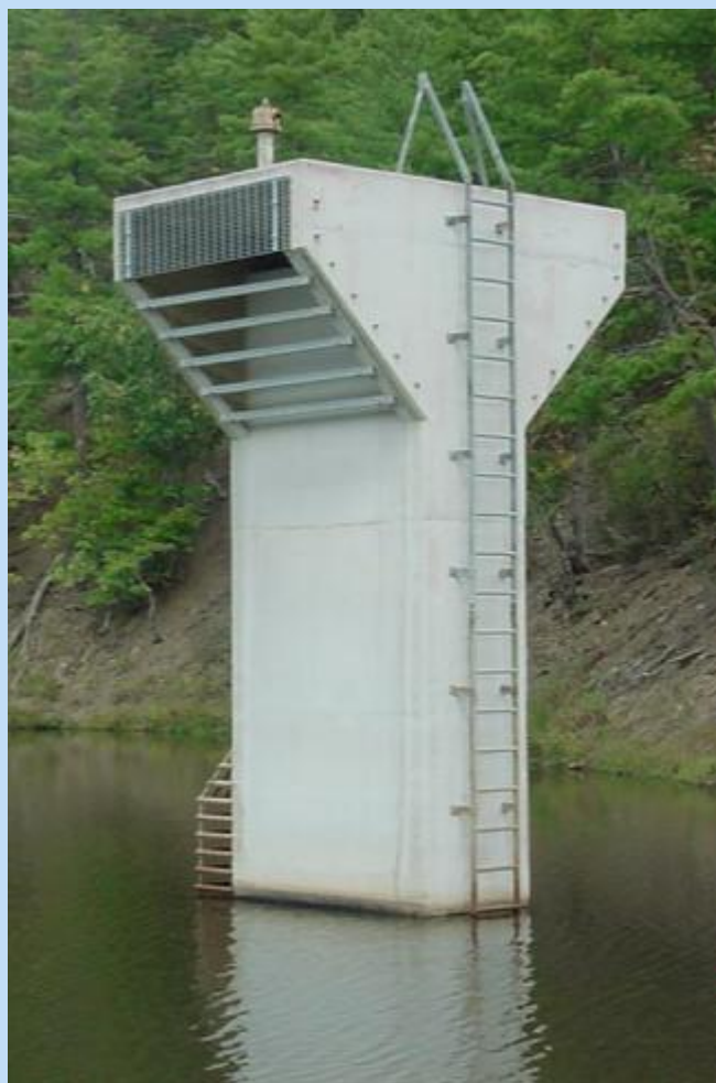
2 Stage Baffled Concrete Riser
