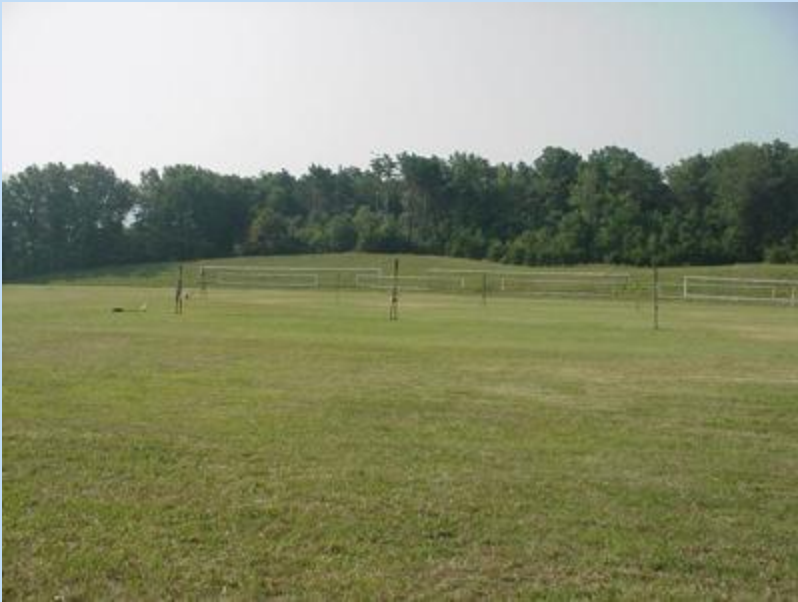
Obstructions in Spillway
