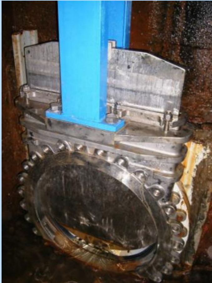
Hydraulically Activated Knife Gate
