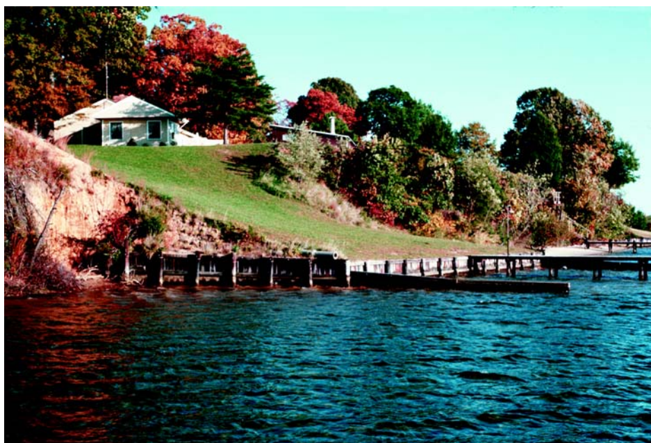
Figure 14A Bulkhead and graded bank.
